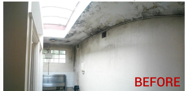
Toilet cubicles before/after
